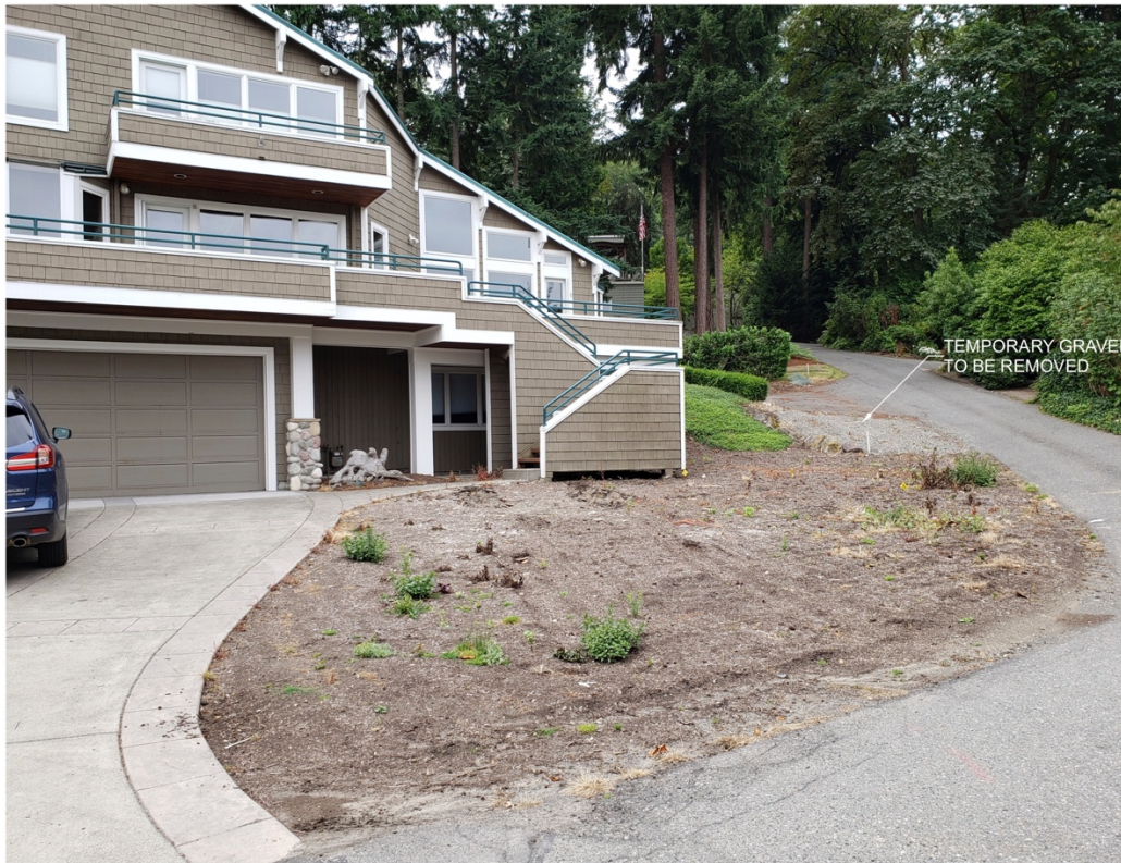
Figure 9 - Temporary gravel has been placed within the piped watercourse buffer. The gravel will be removed and the currently unvegetated portions of the on-site buffer will be planted with native species.
